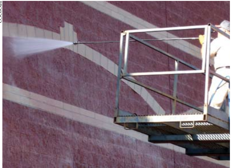
We're not talking garden hose here. Plenty of water, in both the pre-wetting and rinsing steps, is vital to a successful post-construction clean-down of new masonry.
