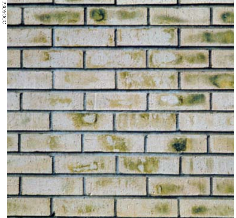
Though muriatic acid is cheaper than appropriate proprietary cleaners, the potential expense in damaged masonry is enormous. Here, improper cleandown with muriatic acid dissolved vanadium salts in the brick, causing ugly green stains.
